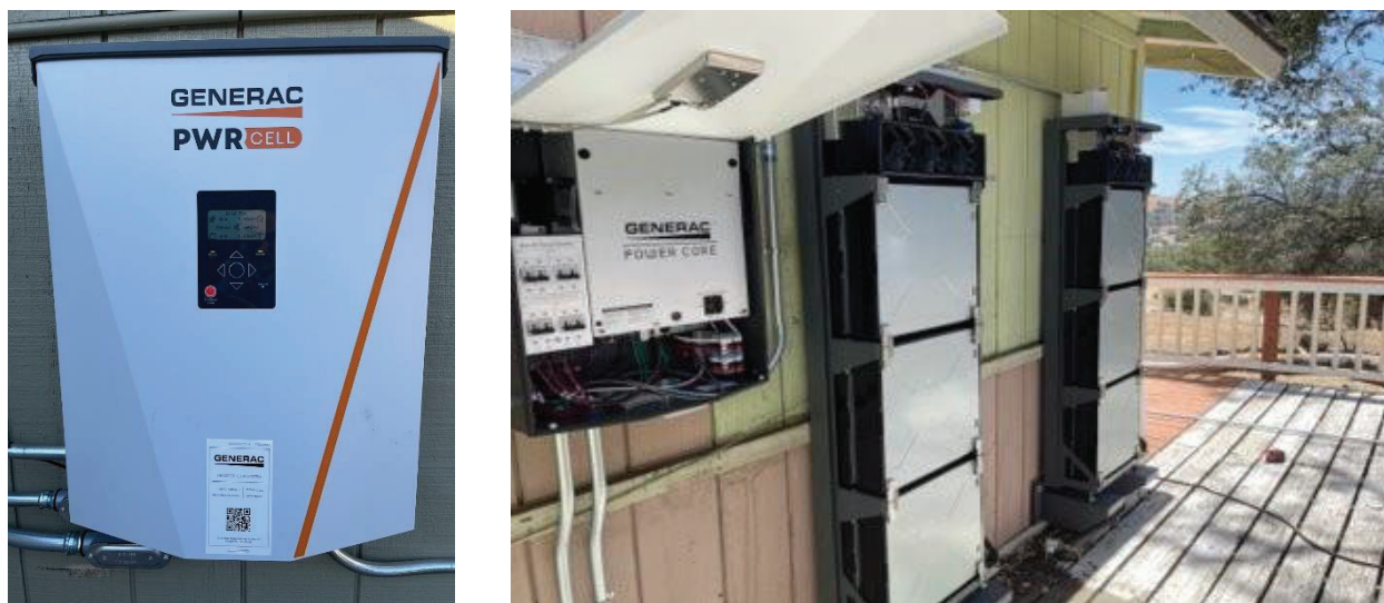
Figure 8-6: FPB Installation at Mobile Home Park Community
