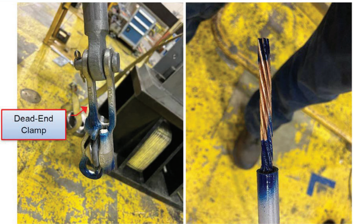
Figure E3. A representative post-test image showing pull-out of the conductor at the dead-end clamp attached to the insulator (north end). 2/0 CU with Type A dead-end shown.
