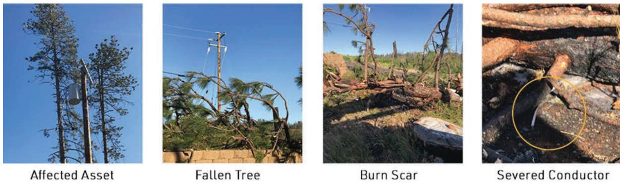
Figure 2: PG&E Covered Conductor Effectiveness – Example 1
