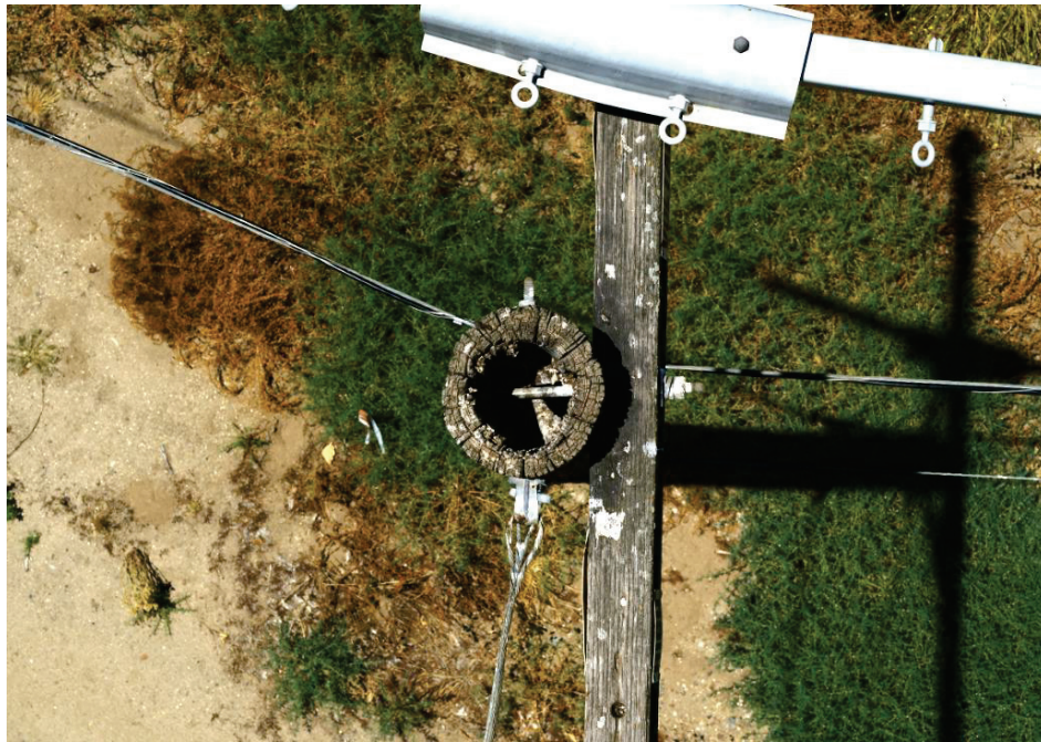
Figure JW-8 Hollow pole top only visible from above
