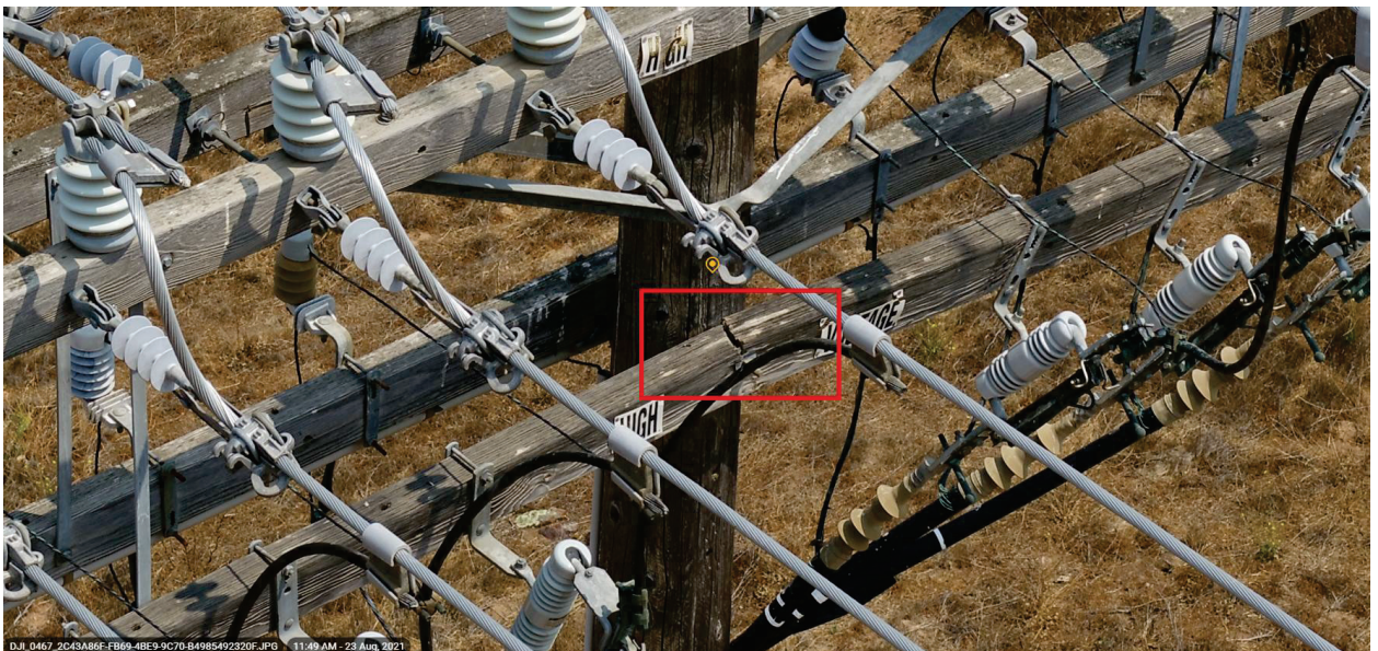
Figure JW-11 Cracked crossarm not visible from the ground
