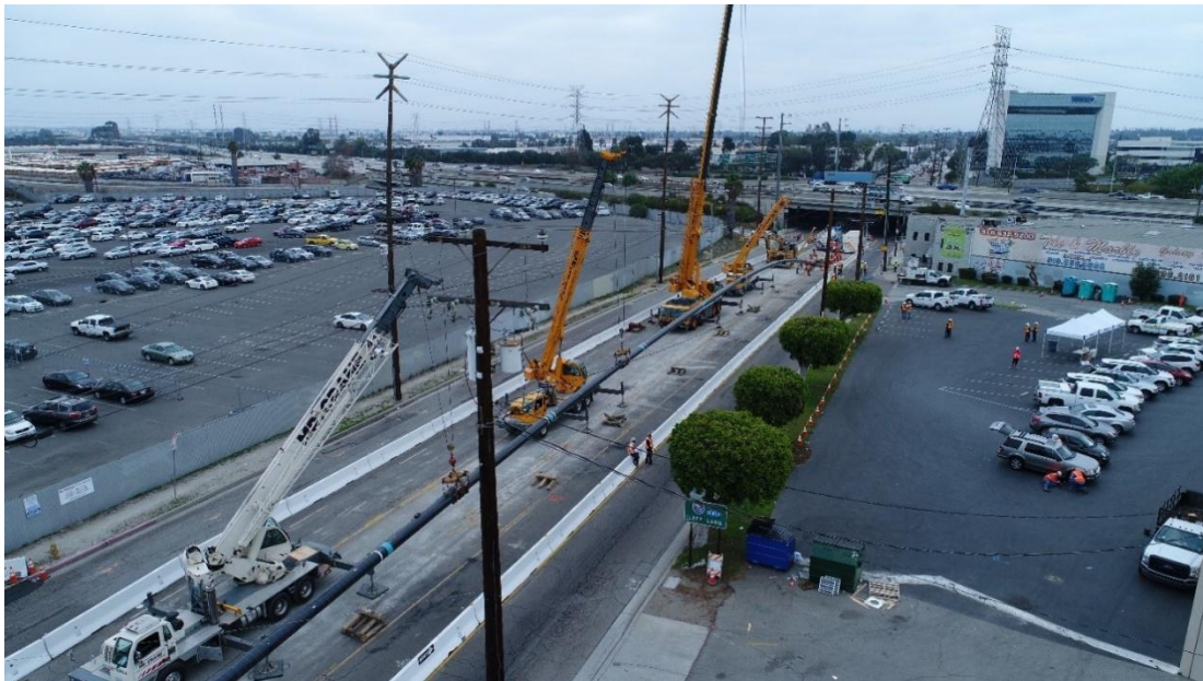
Figure 15: HDD Pullback
