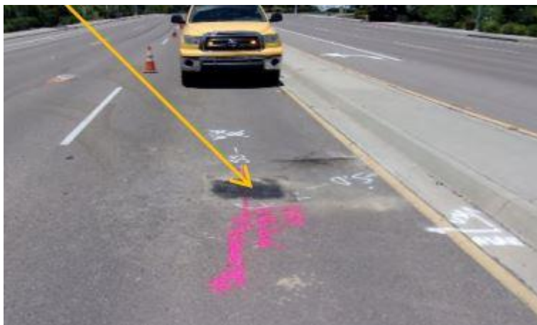
Figure 4: Potholing Location After Restoration
