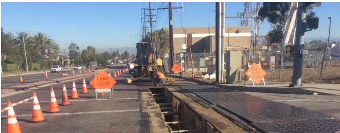
Figure 1: Traffic Control Lane Closure
