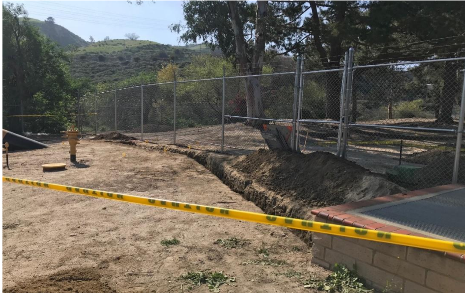
Figure 10: Hand Dug Trench
