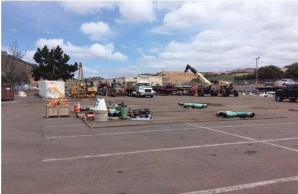
Figure 6: Construction Laydown Yard
