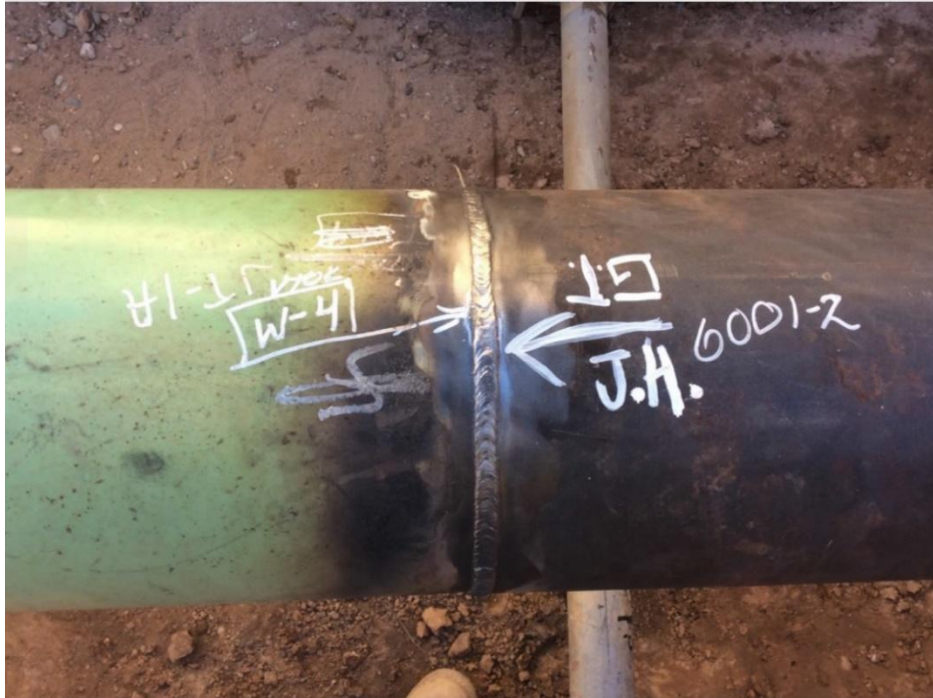
Figure 20: Pipeline Weld
