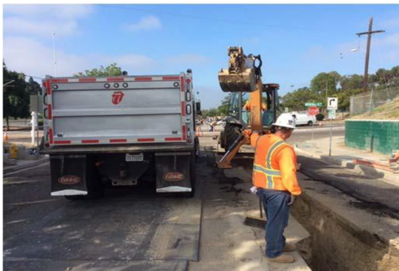
Figure 8: Trench Excavation with Backhoe
