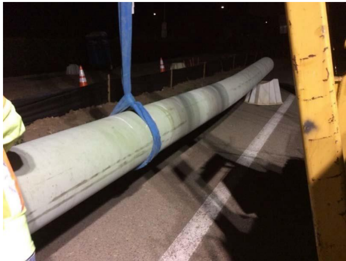
Figure 19: Pipe with Field Bend Laying on Supports
