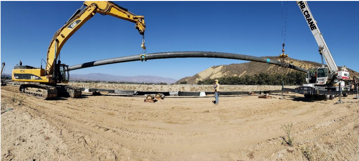
Figure 14: HDD Pullback
