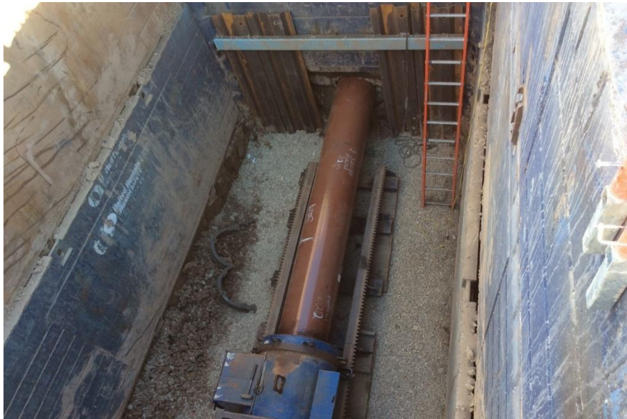
Figure 17: Boring Machine Pushing Casing Pipe
