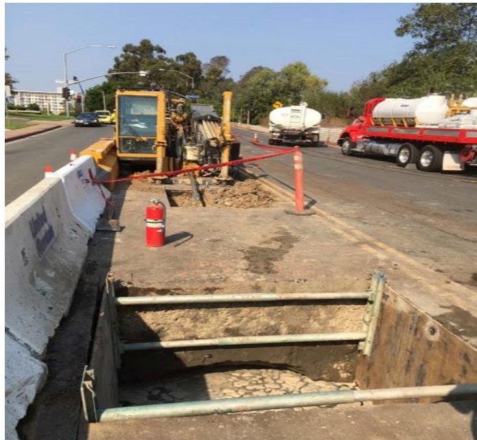
Figure 13: Horizontal Directional Drill (HDD) Equipment
