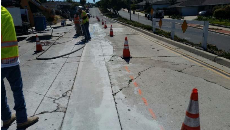
Figure 7: Saw Cutting Trench Pathway
