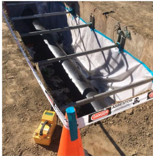
Figure 5: Typical Pipeline Abatement
