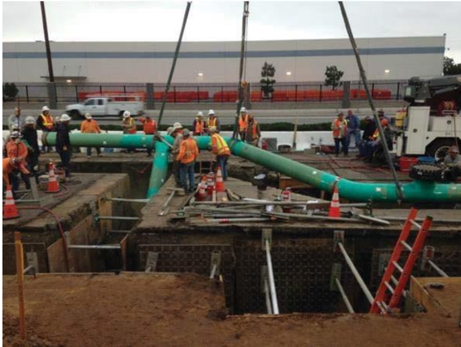
Figure 21: Lowering Section of Pipe into the Trench
