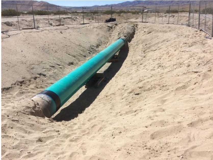
Figure 11: Pipeline Excavation and Repair Site
